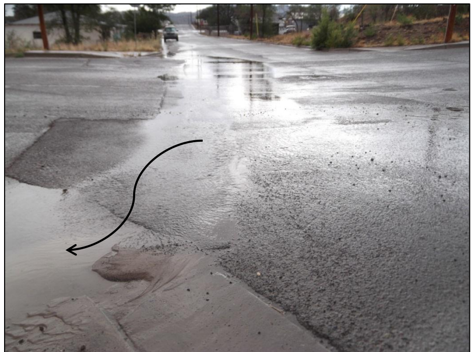
Fig. 3: Street Runoff Flowing Into Detention Basin on July 16, 2013
