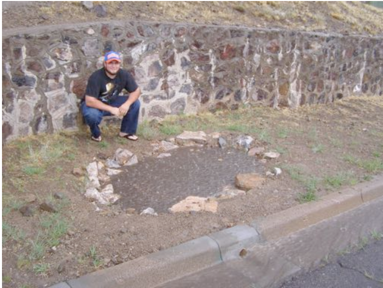
A student at WNMU who came out in the rain to witness the project his class designed and built working perfectly during its first rainstorm, July 11th, 2011
