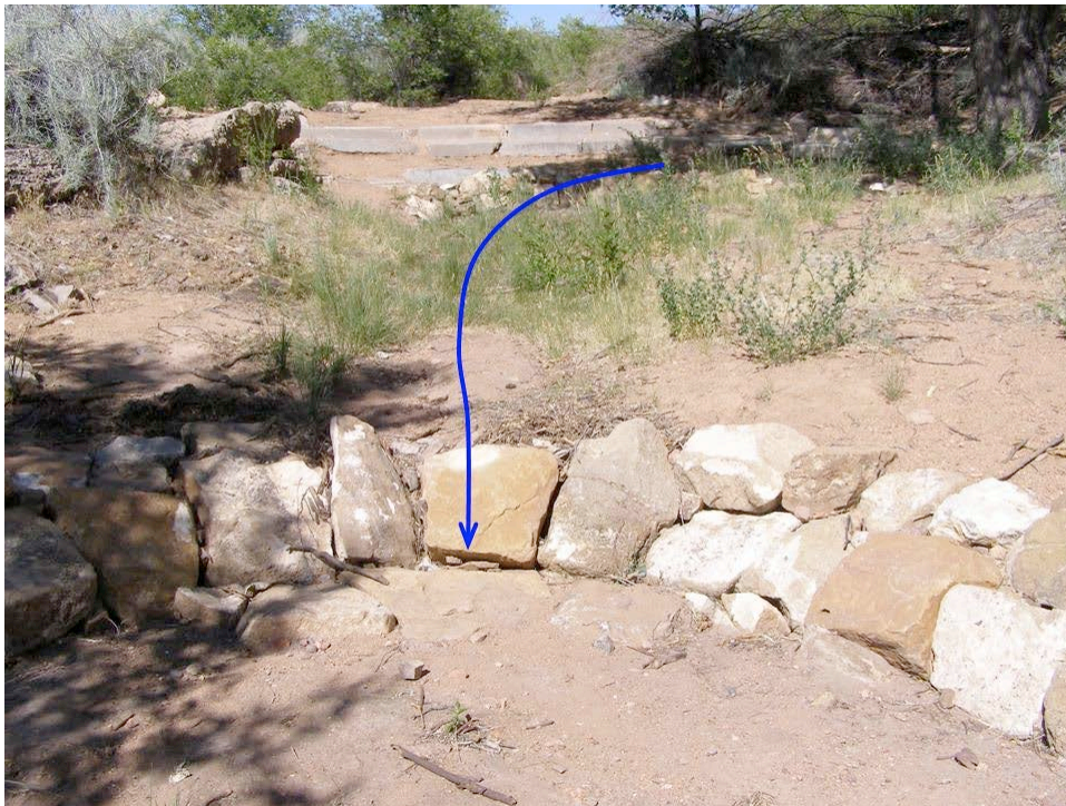
Looking upstream. Overflow from fore-basin goes through two sequences of swale and basin before it is released to the Arroyo Chamisos.
