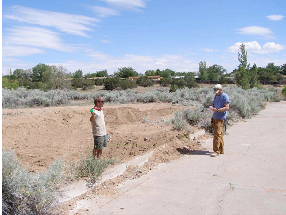
After oxbow basin was excavated, but before curb was cut.
