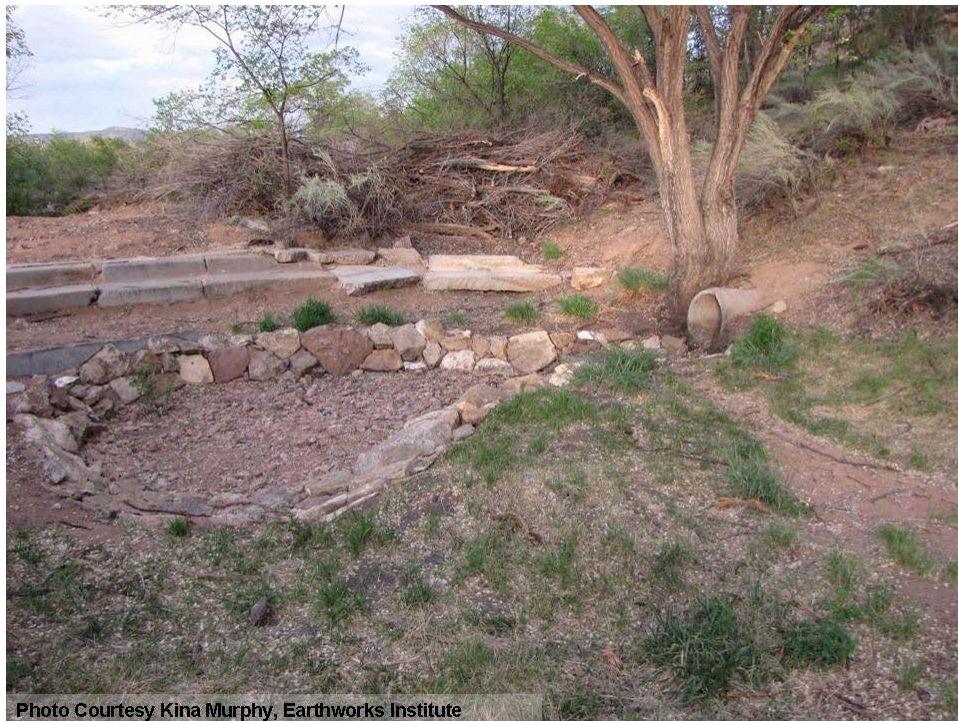
Urbanite site, showing culvert outlet and fore-basin. Photo by Kina Murphy.
