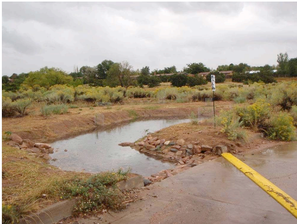
Plastic speed bump was bolted to the drainage channel diagonally to capture all of the base flow, yet allow peak flow to bypass the diversion. Photo by Steve Vrooman.
